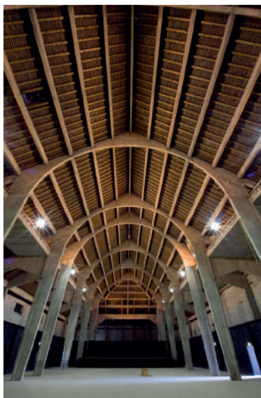
5. West production building in 2001
